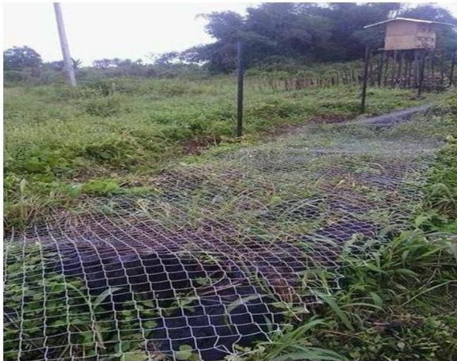
Figure 3. Outlining/ stretching out the wire mesh
