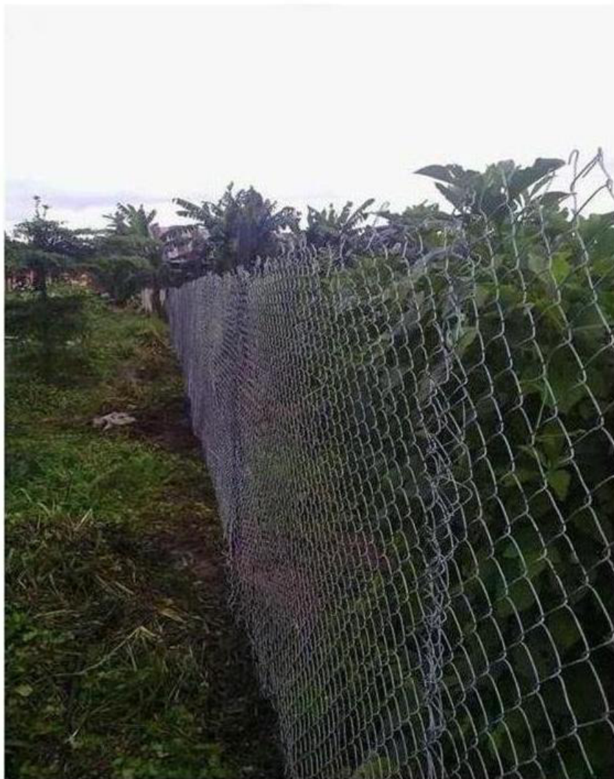
Figure 6. One Side view of constructed fence
