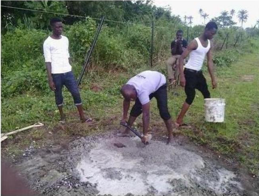
Figure 4. Mixing gravel, sand and cement for casting the fencing posts.
