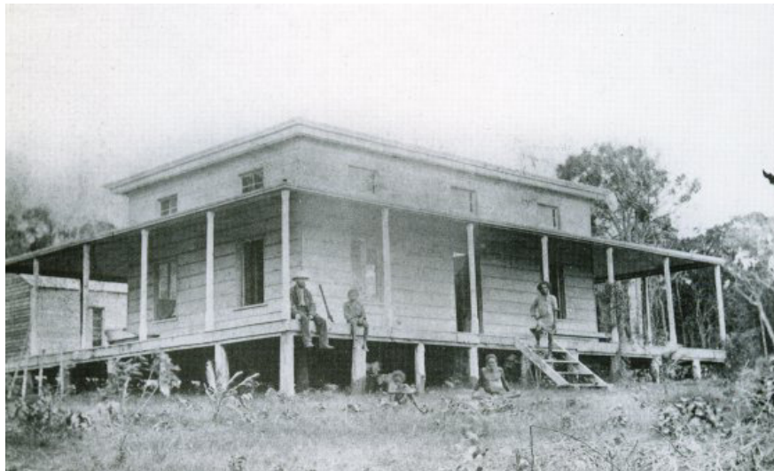
Figure 4. Somerset Hospital c 1868
